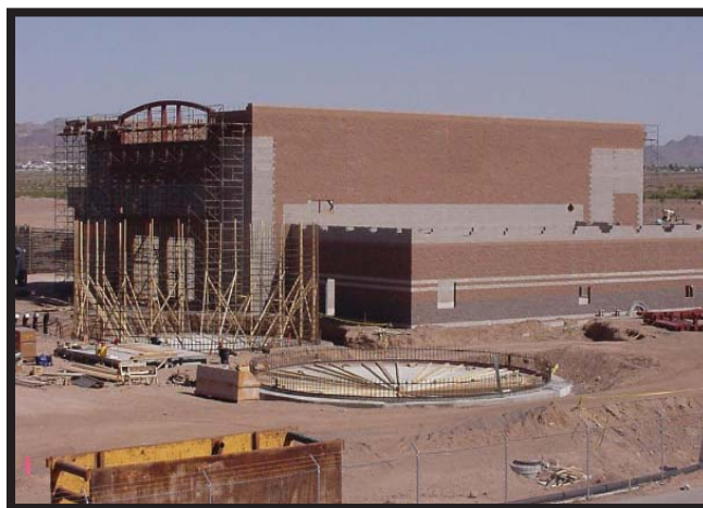
City of Henderson water recycling facility expansion.
