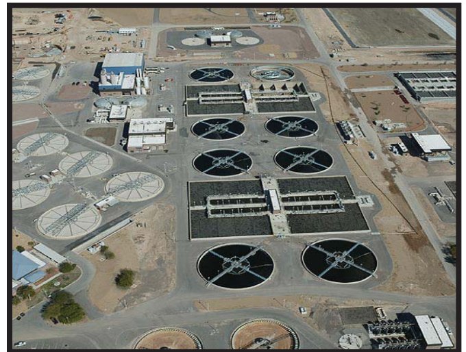
Clark County Water Reclamation District's main treatment facility.
